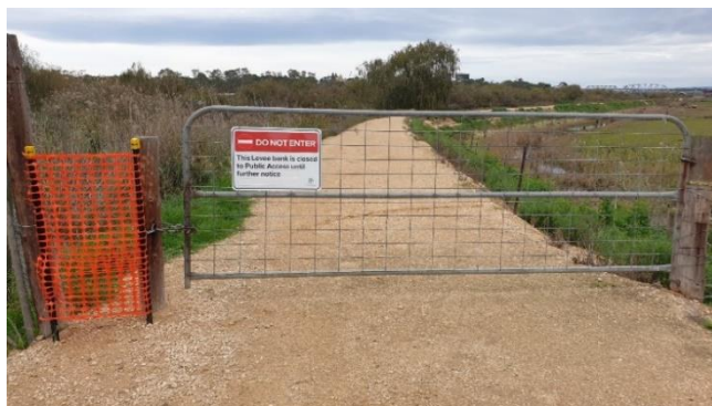
Photo: Restricted access to levee banks.
